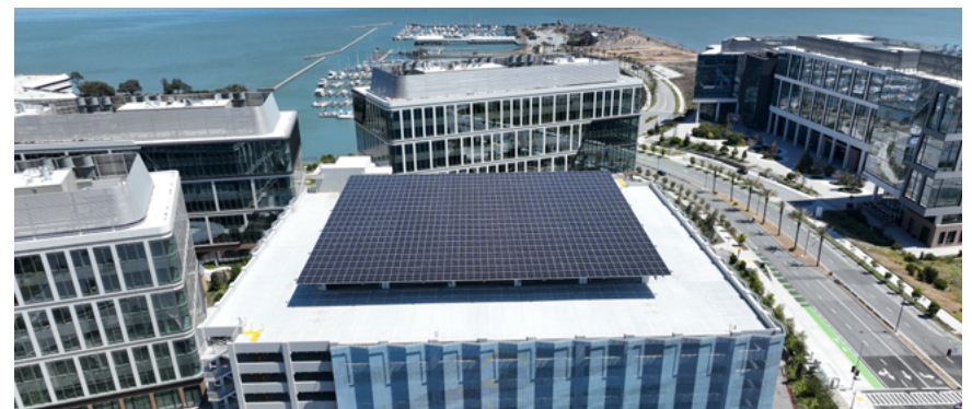
Kilroy Oyster Point Phase 2, South San Francisco, CA — LEED Gold
